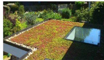
7 Example of a green roof system
